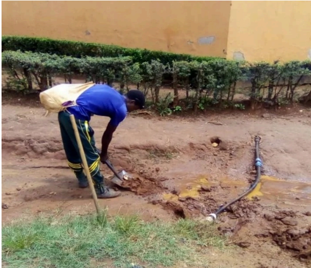
Photo 1: shows the plumber fixing the leakage.
